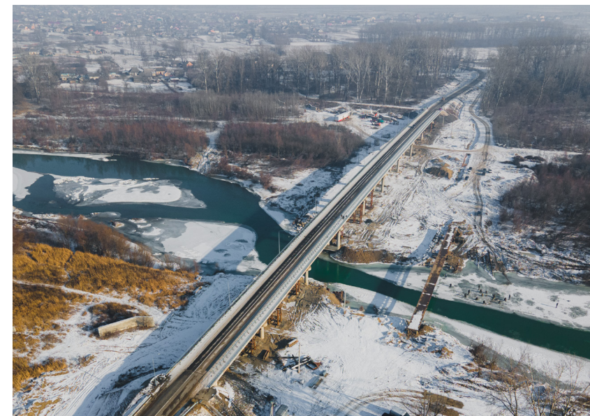
The bridge over the Prut River in the village of Marshintsi, road T-26-06
