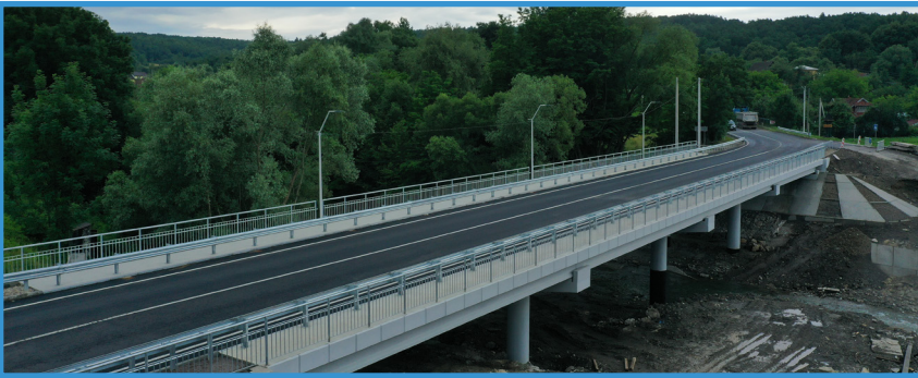
Bridge crossing over the river Lyuchka at km 94+415 of road R-24 Tatariv - Kosiv - Kolomyia - Borshchiv - Kamyanets-Podilsky in the Ivano-Frankivsk region
