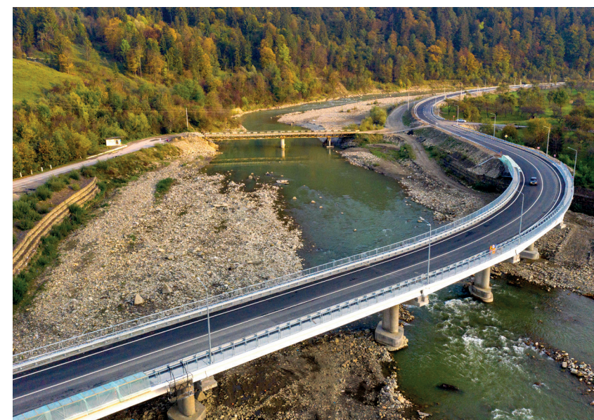
Bridge in Roztoky, Chernivtsi region, road R-62
