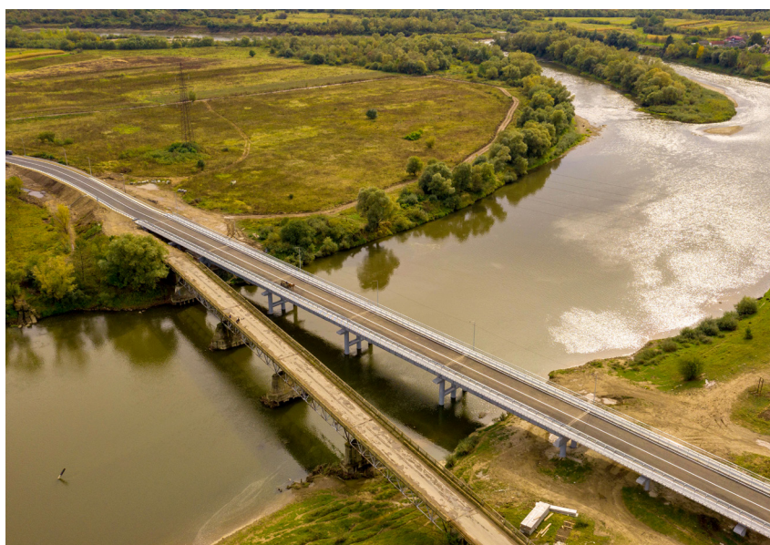
Bridge over the Dniester River, Ivano-Frankivsk region, road T-09-10
