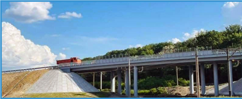
Bridge over the railway at km 164+068 of road N-01 Kyiv - Znamyanka in the Cherkasy region
