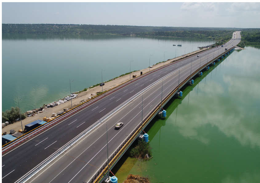
M-05 Kyiv - Odessa - bridge across the Hadjibey estuary at km 445+432 in the Odessa region
